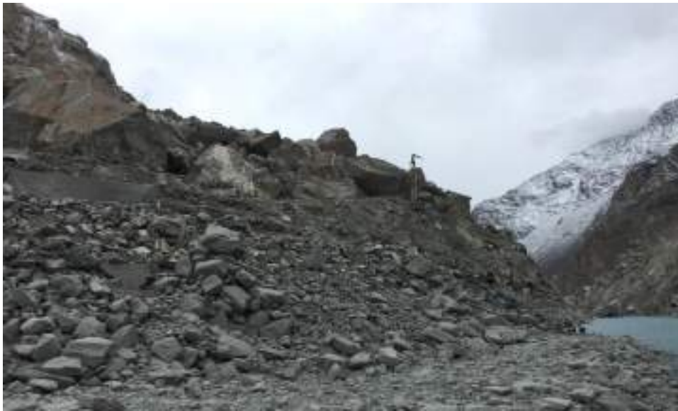
Photo 5-5 Intake Area of Sediment Flushing Channel.
