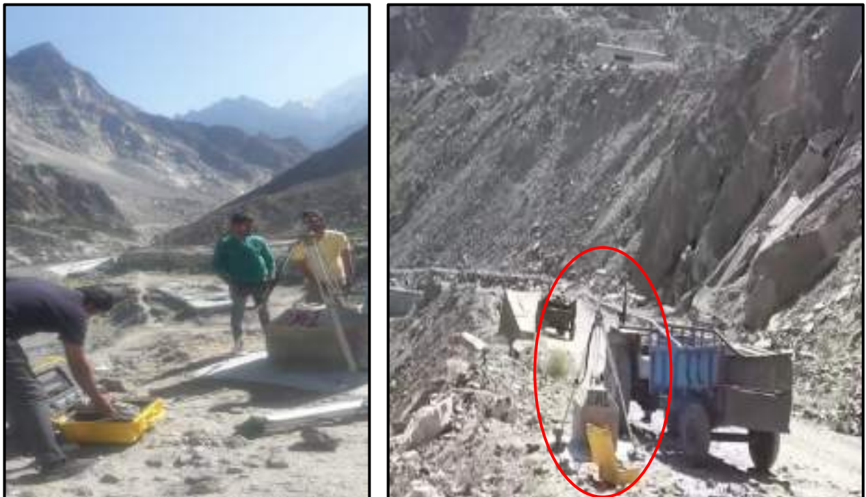
Figure 3-2 Survey of Project's Permanent Reference Benchmark BM-1
