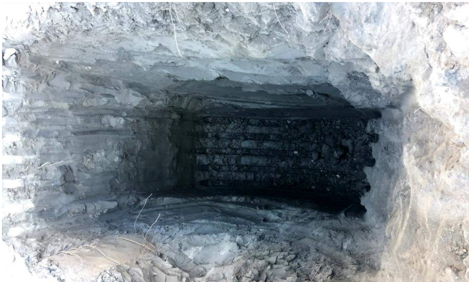
Photo 5-10 TP-3, Excavated for Clayey Silt in P/H area.
