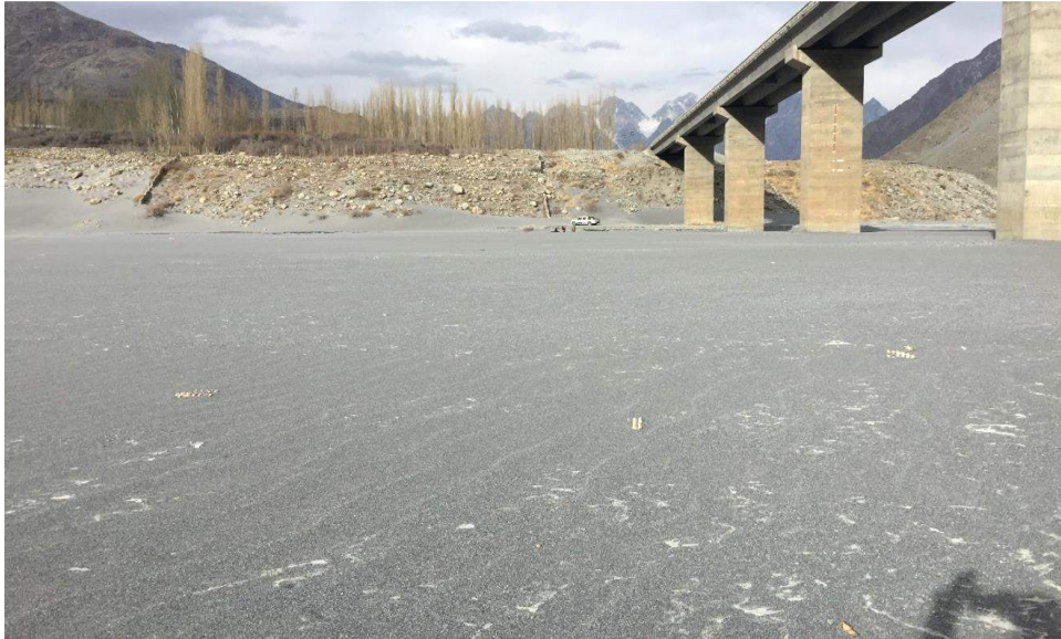
Photo 5-9 Quarry Area Selected for Sand Near Shishkat Bridge.
