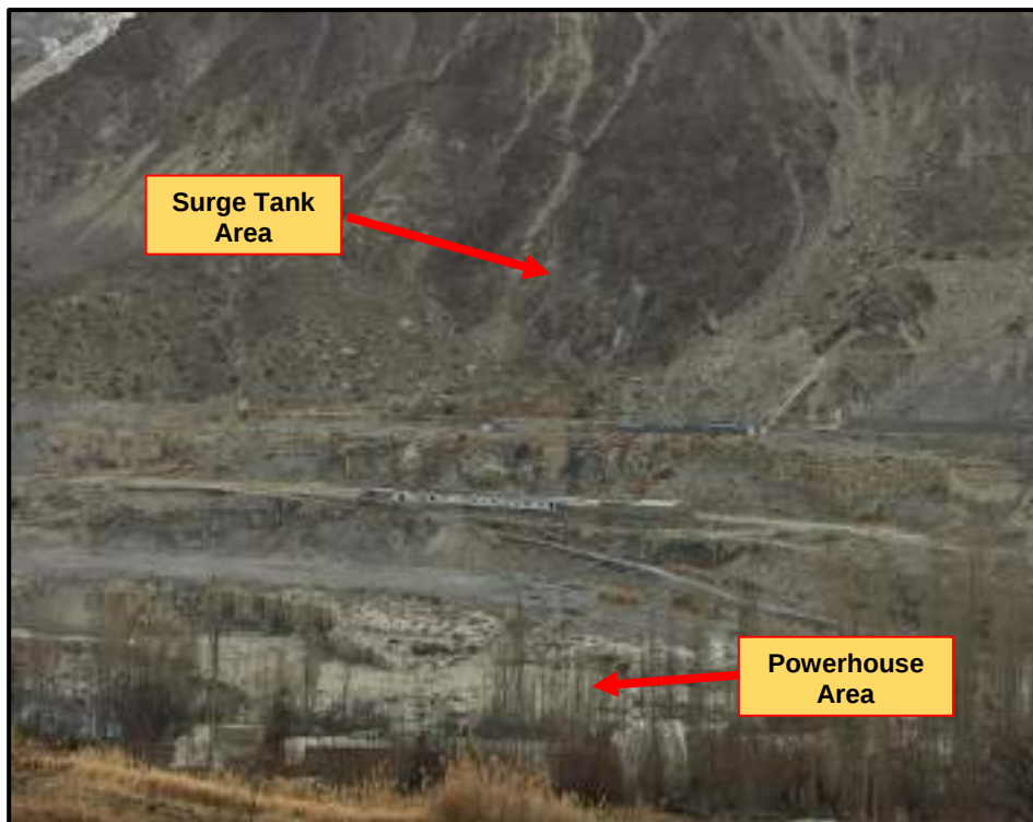
Figure 3.4: A view of Surge Tank and Powerhouse Area
