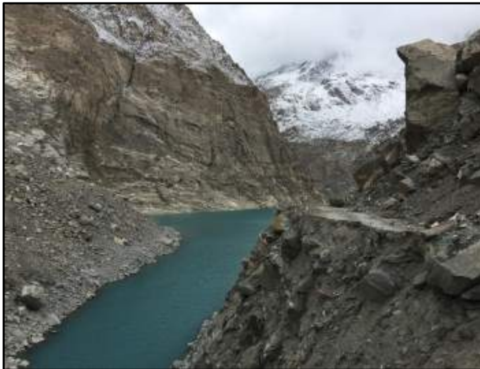
Figure 3.2: Spillway Area (Looking Upstream)
