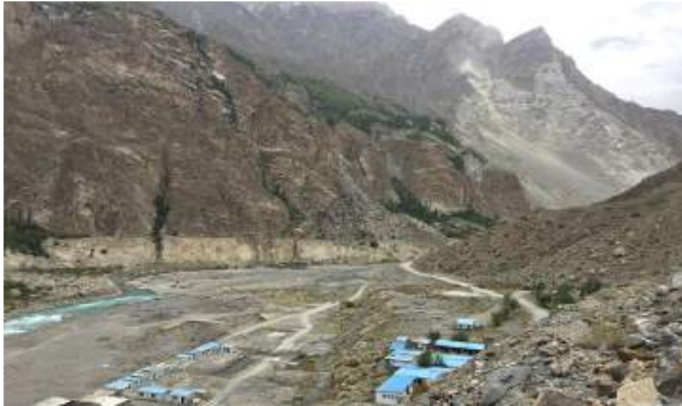
Photo 5-7 Proposed Alignment of Penstock
