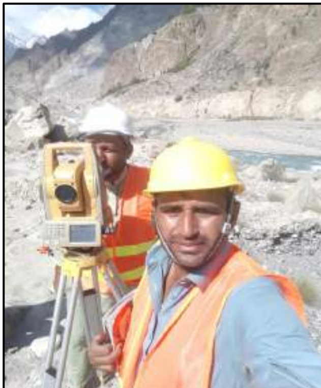
Figure 3-3 Terrestrial Topographic Survey in progress
