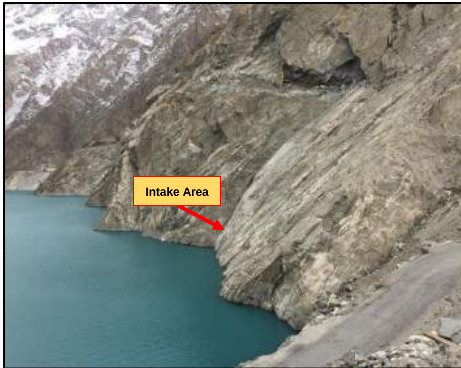
Figure 3.3: A view of Intake Area
