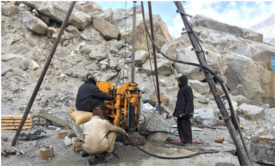
Photo 5-2 Drilling Rig at BH-02 Sediment Flushing Channel
