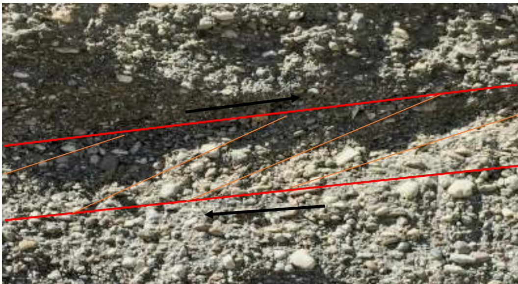
Photo 6-1 Inclined Gravel Layer under Effect of Shearing.
