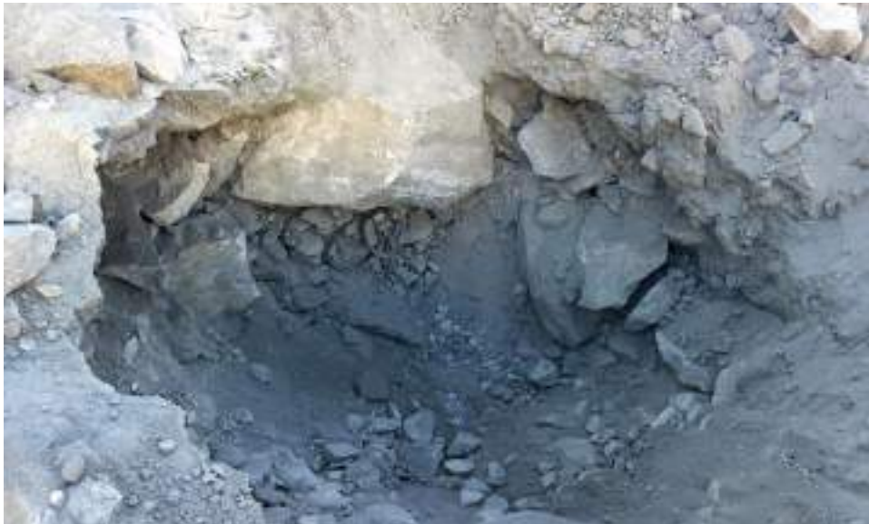
Photo 5-14 View of Slided Mass in TP-6 at Left Side Slope of Hunza River.
