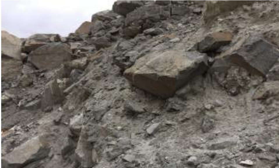
Photo 5-15 Fill Material (Boulder and Gravels) in Slided Mass.
